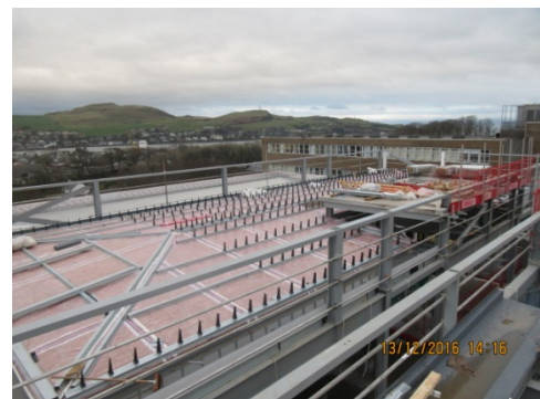
Photograph 2 Roofing contractors progressed onto working on roof grid lines E to G
