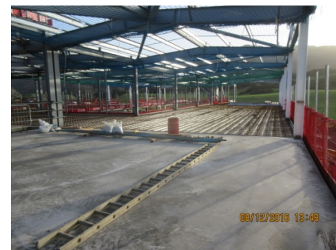
Photograph 4 Concrete slab won 2 nd floor with edge protection in place
