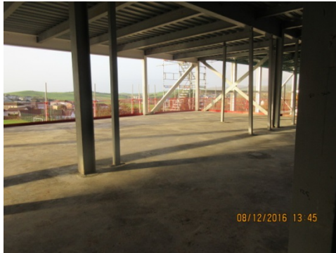
Photograph 5 1st Floor concrete slab complete up to grid point J
