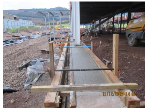
Photograph 10 Concrete placement now in perimeter beam from Grid E to J
