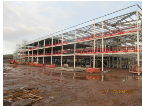
Photograph 8 – West elevation showing the completed structural steelwork from Grid A to U
