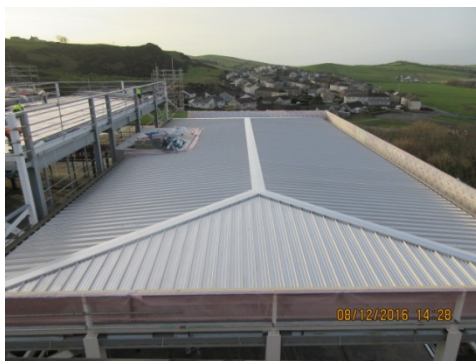
Photograph 1 Sports Hall Roof Complete
